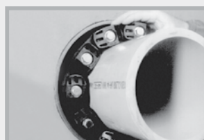
Push MASTER-SEAL into the annular gap
