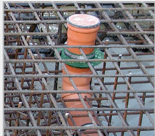
The RONDO, shortly before placement of concrete. The drainpipes are securely and permanently sealed against rising moisture.
