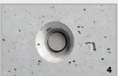
4 Flush seal for distance tubes with cone.
