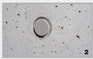
2 Sealing of distance tube with lip
