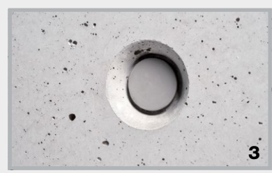
3 Sealing of distance tube with cone
