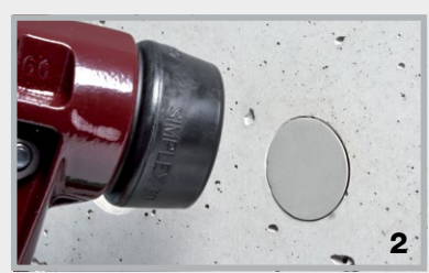
2 Drive in with rubber mallet
