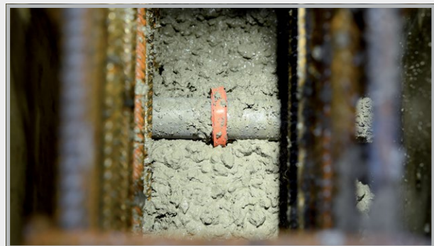
At the construction site
