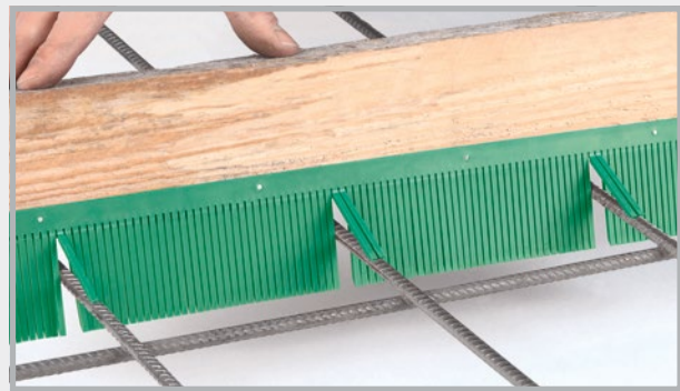
Position, align and anchor back the square timber
