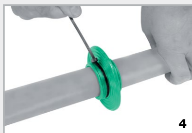
Tighten both fastening straps by hand
