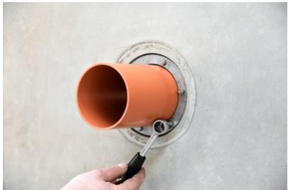
Tighten the screws crosswise through one turn.
