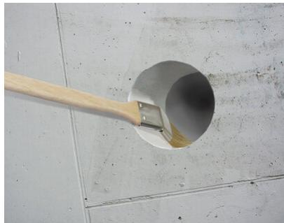
When installing a **MASTER-RING** gasket insert in a core drill hole the inside of the core drill hole has to be preserved with an epoxy resin ( PROTECT EP resin).
