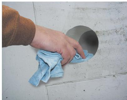
Before installation the **MASTER-RING** gasket insert, the inside of the core drill hole and the outside of the gas, water, sewage pipes as well as the cables have to be cleaned.
