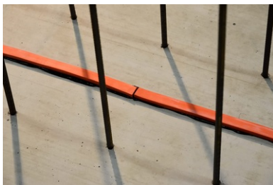
Straight butt joint
