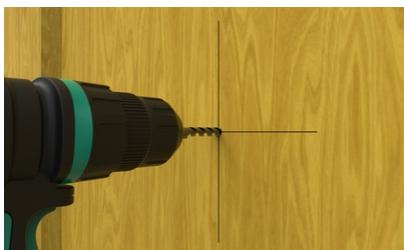
Mark the position of the pipe on the formwok and drill an Ø8mm hole in the center.
