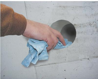
Before installing the **MASTER-SEAL** modular seal, the inside of the core drill hole and the outside of the gas, water, sewage pipes as well as the cables have to be cleaned.
