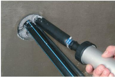
Fill the duct completely with **FLEX 2000**.
