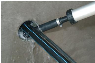
Insert the flexible nozzle into the duct and seal it with **FLEX 2000** starting from the securing block.
