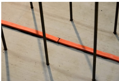
Straight butt joint
