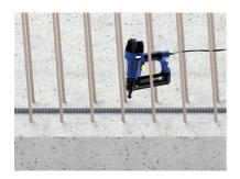
The distance between nails should not exceed 25 cm in the longitudinal direction of the swelling tape. At the beginning of the tape and if tape sections are used, pull back the protective sheating approx. 5 cm, cut off the swelling tape and fold over the extra length of sheating to prevent contact with water.
