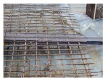
The **stopend panel joint sheet metal ABS** is positioned between the lower and upper reinforcement layer (foundation – foundation area) or the outer and inner reinforcement layer (wall – wall area). The perforated plate is fastened to the reinforcement using
