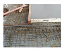
In the second concrete segment, as soon as the protective foil has been removed immediately before concreting, concrete can be placed directly against the stopend panel joint sheet metal ABS.
