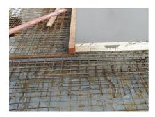
In the second concrete segment, as soon as the protective foil has been removed immediately before concreting, concrete can be placed directly against the stopend panel joint sheet metal ABS.
