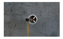
After that, the **FIX formwork aid** can be pushed out.
