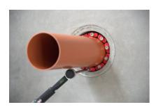
Tighten the screws clockwise one after the other with a torque wrench.
