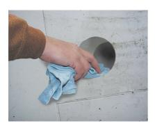
Before installing the **MASTER-SEAL** modular seal, the inside of the core drill hole and the outside of the gas, water, sewage pipes as well as the cables have to be cleaned. The medium pipes / cables must be dimensionally stable in the sealing area and must not be damaged.
