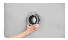
Insert the **MASTER-RING** gasket insert into the lining pipe or the perserved core drill hole and push the pipe/cable through.
