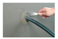
Close the duct with fast-curing cement and smooth it flush with the surface.
