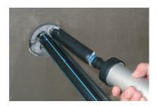
Fill the duct completely with FLEX 2000.
