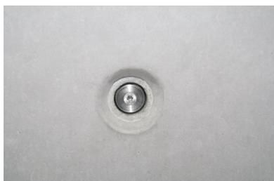
**STOPPER SCREW type in** mounted in tie point with flush seal.
