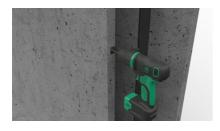
The wall formwork is drilled in order to fix the mounting bracket.
