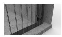
The overlapping area on the floor/wall joint sheet metal is secured with two fixing clips.
