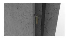
The mounting bracket is fixed with a drive-in plug.
