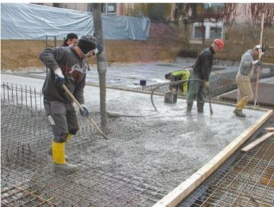
Before the segment is concreted, the protective foil must be removed from the joint sheet metal.
