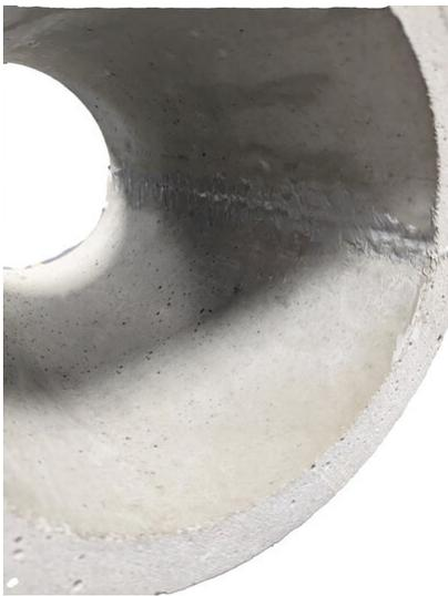
Smooth out the joints inside the casing to obtain a clean surface for the possible installation of a gasket insert or similar.
