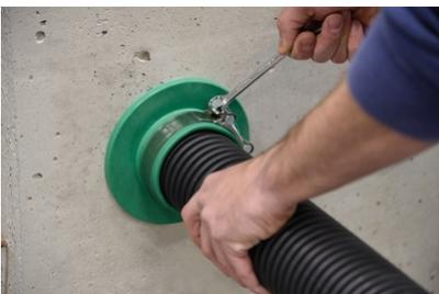
Secure the pipe by hand-tightening the clamp.
