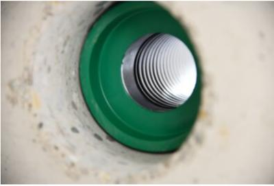
The corrugated pipe is now connected water pressure-tight to the core drilling / lining pipe.
