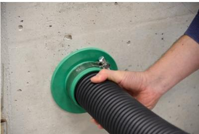
Then place the clamp over the connection seal and push the media pipe in as far as it reaches the stop.
