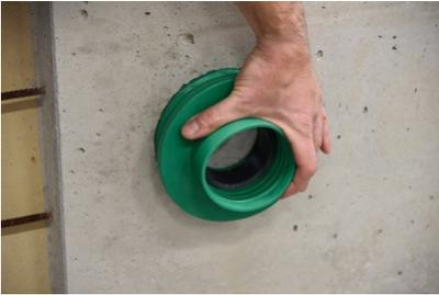
The **Connector connection seal** is positioned in the core drilling / lining pipe.
