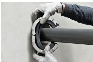
Place the **MASTER-Ring Multi split version** around the installed pipe.
