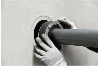
Close the gasket and reinstall the locking clip and close it as well.
