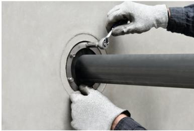
Tighten the screws crosswise through one turn.
