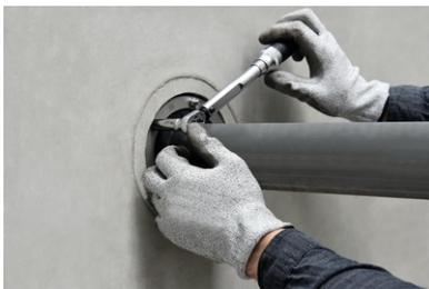
Tighten the screws to the specified max. torque. ( $\emptyset$  100/150/200 = 5Nm;  $\emptyset$ 250 = 10Nm).
