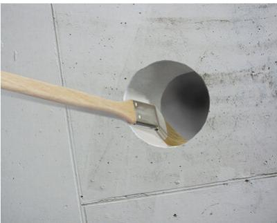
When installing a **MASTER-RING** gasket insert in a core drill hole the inside of the core drill hole has to be preserved with an epoxy resin ( PROTECT EP resin).
