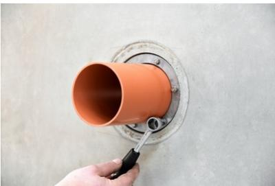
Tighten the screws crosswise through one turn.
