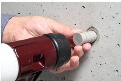
The **STOPPER mini 22** is installed by driving it in with a hard rubber mallet (weight 1500 - 2000 g) using reasonable force.
