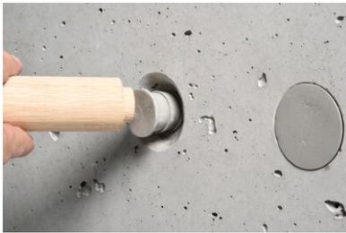
If used with a tapered cone, the last bit of the **STOPPER mini 22** must be driven into position using a drive-in aid.
