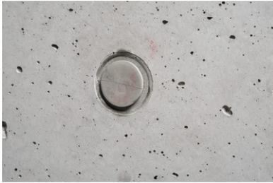
If a lip is used, the **STOPPER mini 22** must be driven in so that it is flush.
