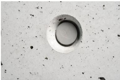
The **STOPPER mini 22** is then driven in so far that the small surrounding edge is resting against the inner concrete surface.
