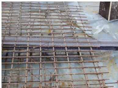
The **stopend panel joint sheet metal ABS** is positioned between the lower and upper reinforcement layer (foundation – foundation area) or the outer and inner reinforcement layer (wall – wall area).
