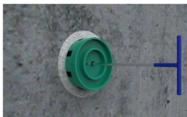
After removing the formwork, the formwork **FIX formwork aid** can be pulled out by using the **FIX removal aid** and the screw can be removed from the pipe.
