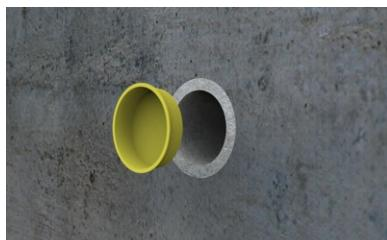
After setting up the finished wall part, the construction period cover is removed first (if installed)
