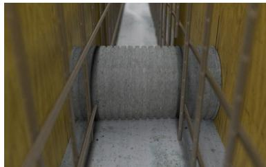
The reinforcement can then be laid, the second formwork placed and the wall concreted.
