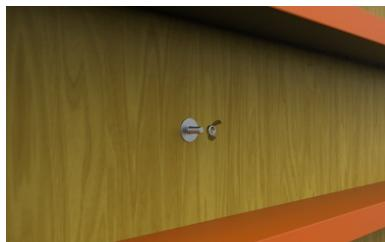
After concreting, the wingnut and washer are removed and set aside.
