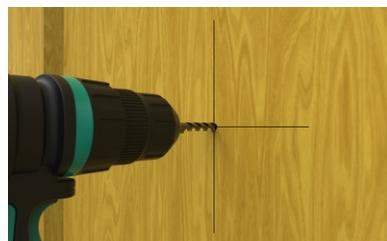
Mark the position of the pipe on the formwok and drill an Ø8mm hole in the center.
