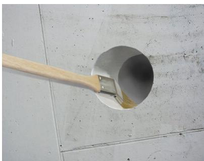
When installing a **MASTER-SEAL** modular seal in a core drill hole, the inside of the core drill hole has to be preserved with an epoxy resin (PROTECT EP resin). The preservation serves to obtain a smooth surface and also as protection of the cut reinforcement steels against corrosion.
