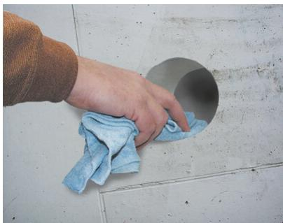
Before installing the **MASTER-SEAL** modular seal, the inside of the core drill hole and the outside of the gas, water, sewage pipes as well as the cables have to be cleaned. The medium pipes / cables must be dimensionally stable in the sealing area and must not be damaged.
