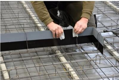
Overlap the **VB JGS joint sheet metal** by at least 6 cm and press the two ends firmly together. The joint must be glued over its full height and entire surface to prevent subsequent water permeation. There must be no contamination on the adhesive surfaces that could interfere with bonding.
