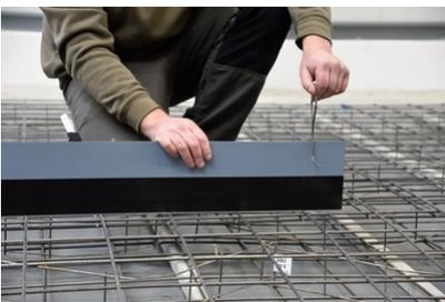
Place the **VB JGS joint sheet metal** in the centre of the rising wall on top of the upper reinforcement layer. Push the mounting brackets with a maximum distance of 70 cm over the sheet metal and fix them to the upper reinforcement layer with binding wire.
