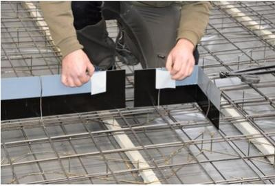
To do so, the upper protective foil must be turned back in the area subsequently to be joined.
