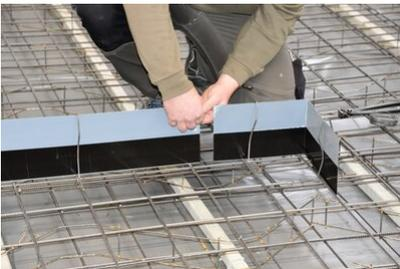
The **VB JGS joint sheet metal** must overlap by at least 6 cm in the area of the joint, in the straight sections and also in the corner area.
