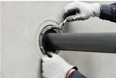
Tighten the screws crosswise through one turn.
