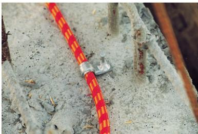
The hose can be fastened in place with metal clips for nailing (manual or nail gun).
