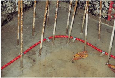
All changes in direction must be implemented with a sufficiently wide bending radius in order not to damage the hose/restrict the overall injection flow.
