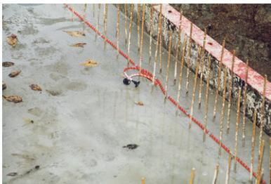
Place the hose centrally in the construction joint, within the reinforcement.
