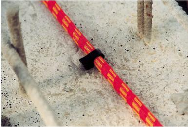
Alternatively, the hose can be fastened in place with plastic clips, either set in the fresh concrete or subsequently hammered into an 8 mm drill hole. The distance between the fastening clips must not exceed 15 cm. The hose must be in continuous contact with the concrete and must not be allowed to float.
