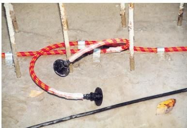
Successive injection hose sections must overlap by at least 20 cm in order to ensure continuous injection of the joint.
