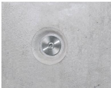
**STOPPER SCREW type covered** mounted in tie point with cone.
