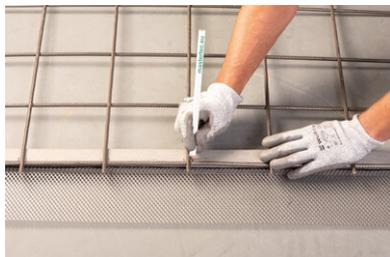
The position of the reinforcement must be marked on the ABS spacer
