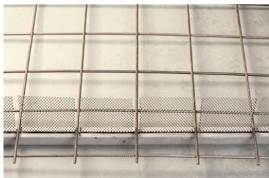
Then place the **ABS spacer "Flex"** in the desired position and place the reinforcement mat.
