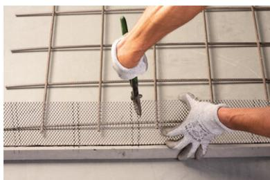
Then use tin snips or other suitable tool to cut into the rib lath along the markings.
