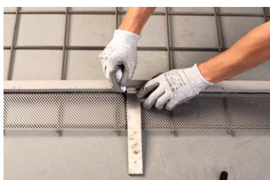
Use a ruler or angle to mark the position of the reinforcement on the rib lath.
