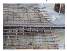
The **stopend panel joint sheet metal ABS** is positioned between the lower and upper reinforcement layer (foundation – foundation area) or the outer and inner reinforcement layer (wall – wall area).
