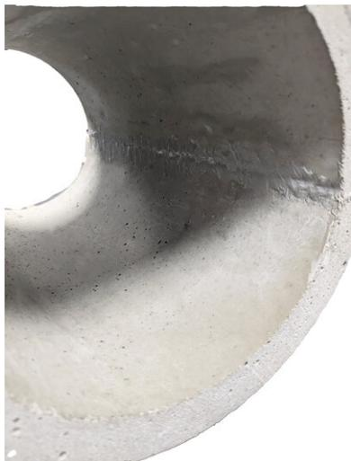
Smooth out the joints inside the casing to obtain a clean surface for the possible installation of a gasket insert or similar.
