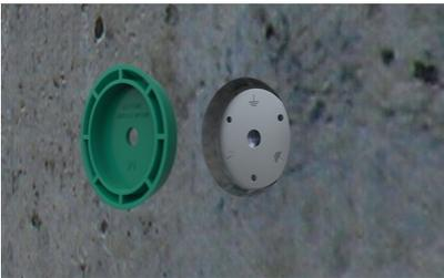
Finally, remove the **FIX EFP formwork aid**.
