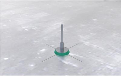
Apply the fixed earthing terminal to the intended position on the steel formwork.
