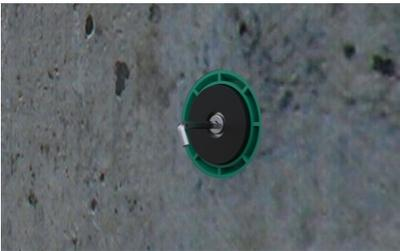
After removing the formwork, loose the screw with an allen key and remove the **FIX Magnet** from the formwork aid.
