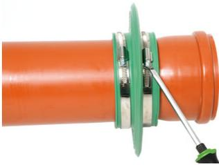
Apply lubricant to the clamping range of the strap, then tighten the clamping straps sufficiently using a screwdriver to prevent the **RONDO sealing collar** from shifting.
