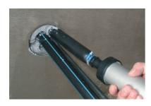
Fill the duct completely with **FLEX 2000**.
