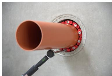
Tighten the screws clockwise one after the other with a torque wrench.
