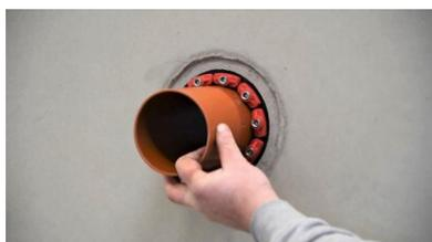
Push the **MASTER-SEAL** modular seal over the medium pipe, insert both into the preserved core drill hole and position the **MASTER-SEAL** modular seal appropriately. The **MASTER-SEAL** modular seal must be installed as close as possible to the outside of the wall ( earth-side, water-side).
