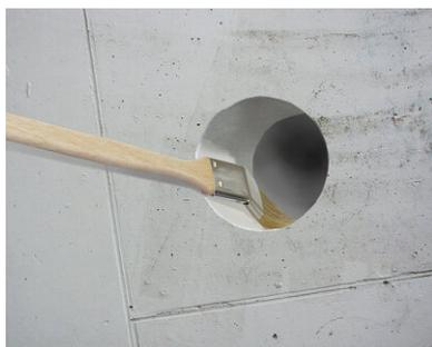
When installing a **MASTER-SEAL** modular seal in a core drill hole, the inside of the core drill hole has to be preserved with an epoxy resin (PROTECT EP resin).
