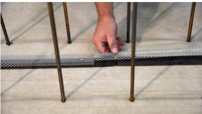
In the case of butt joints in the straight line and the use of swelling tape grids, the joints of swelling tape and swelling tape grid should be offset.
