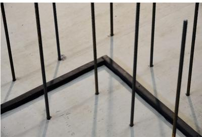
Both, straight and angle joints need to be butt jointed.
