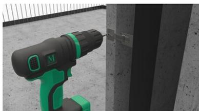
The wall formwork is drilled in order to fix the mounting bracket.
