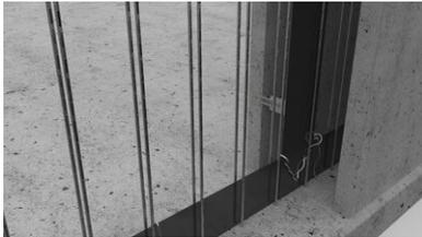
The overlapping area on the floor/wall joint sheet metal is secured with two fixing clips.
