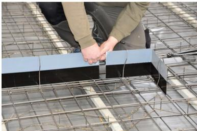
The **VB joint sheet metal** must overlap by at least 6 cm in the area of the joint, in the straight sections and also in the corner area.
