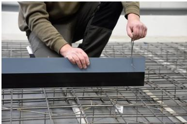
Place the **VB joint sheet metal** in the centre of the rising wall on top of the upper reinforcement layer.
