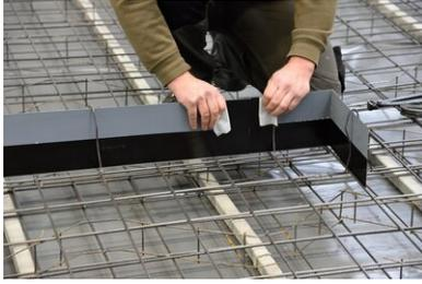
Overlap the **VB joint sheet metal** by at least 6 cm and press the two ends firmly together. The joint must be glued over its full height and entire surface to prevent subsequent water permeation. There must be no contamination on the adhesive surfaces that could interfere with bonding.
