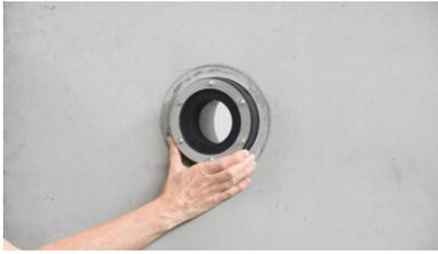
Insert the **MASTER-RING** gasket insert into the lining pipe or the preserved core drill hole and push the pipe/cable through.
