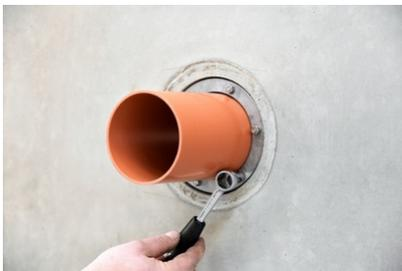
Tighten the screws crosswise through one turn.
