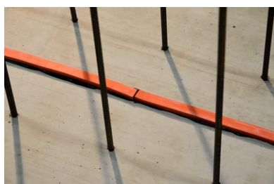
Straight butt joint
