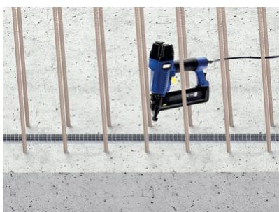
The distance between nails should not exceed 25 cm in the longitudinal direction of the swelling tape. At the beginning of the tape and if tape sections are used, pull back the protective sheathing approx. 5 cm, cut off the swelling tape and fold over the extra length of sheathing to prevent contact with water.
