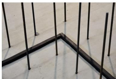
Both, straight and angle joints need to be butt jointed. The joint areas must be form-fit in order to avoid any discontinuity in the system.
