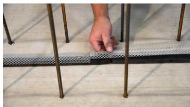
In the case of butt joints in the straight line and the use of swelling tape grids, the joints of swelling tape and swelling tape grid should be offset.
