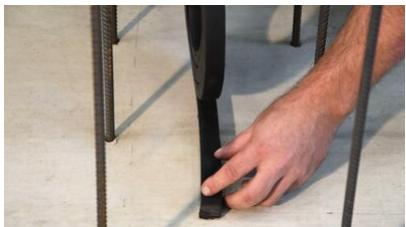
Once the swelling tape adhesive has been applied in the centre of the joint, the **MASTERSTOP bentonite swelling tape** is placed on the adhesive and gently pressed on, moving it slightly back and forth, crosswise to the longitudinal axis.
