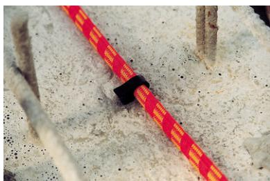
Alternatively, the hose can be fastened in place with plastic clips, either set in the fresh concrete or subsequently hammered into an 8 mm drill hole.
